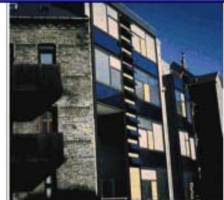
... and after renovation
