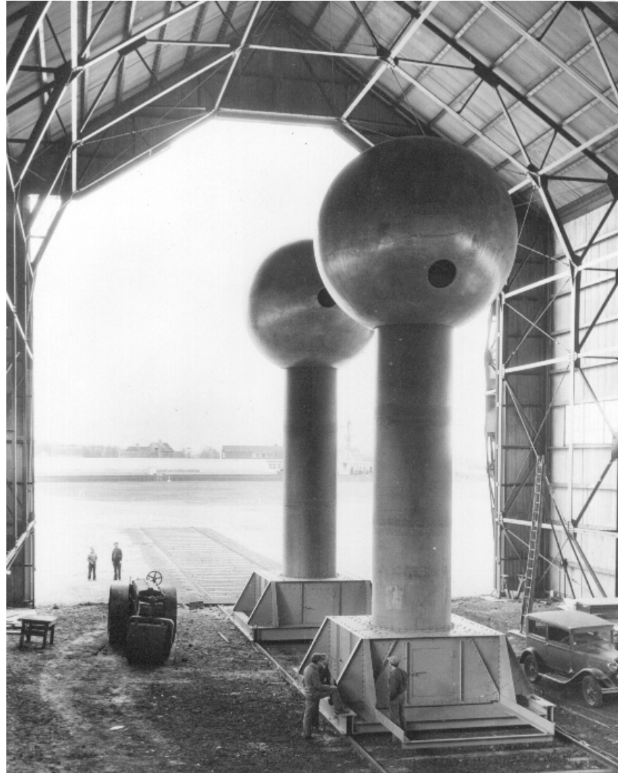
THE GENERATOR IN THE HANGAR AT ROUND HILL
