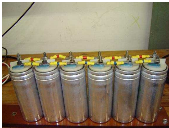
Figure 31: Prototype capacitor bank with capacitors connected in parallel using crimped 6mm wire.
