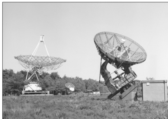
Figure 16: The telescopes at Dwingeloo Observatory, with the western Würzburg in the right foreground. The equatorial mounting can be seen clearly. The 25-m telescope is on the left, and the eastern Würzburg can be seen in the distance (photo by H. Schneider).
